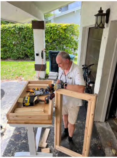
Carefully assembling the face frame.
