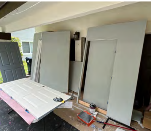
All doors were "pre-hung" with removable stringers to help speed setup.
