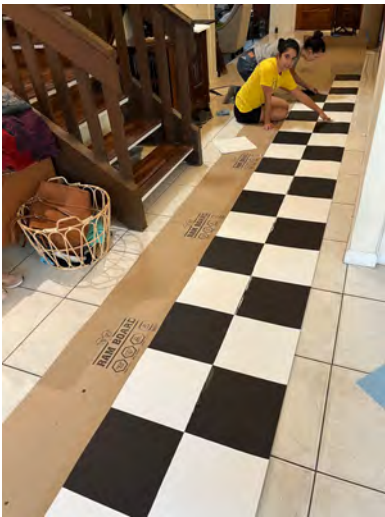
Each run of rollable flooring were 30' x 3' tiles giving us a set of 5 runs.
