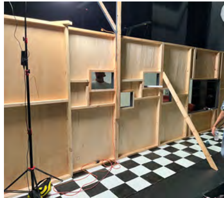
The front wall only needed one support.
